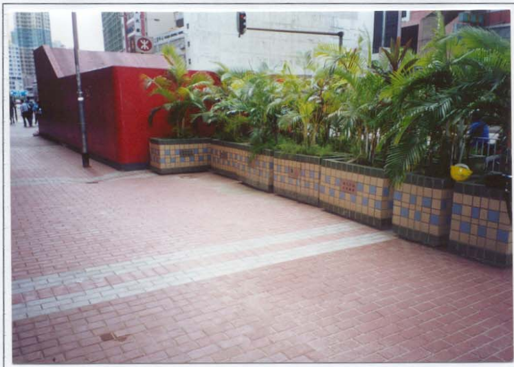
Comparison of recycled aggregate pavers(pink colour) with Correctional Services Department's pavers(red colour).
